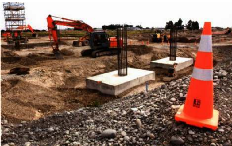
Pier construction at the Aidanfield Underpass.
